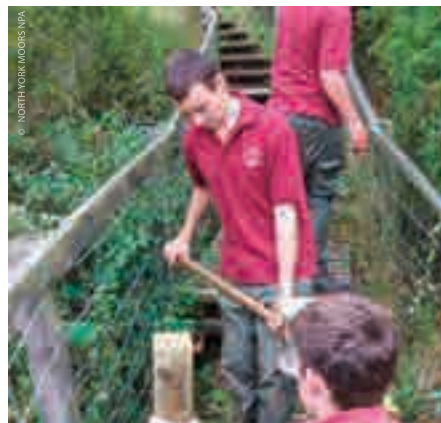
North York Moors apprentices construct a boardwalk
