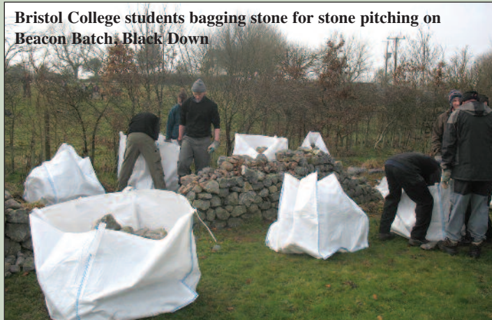
Beacon Batch stone pitching
